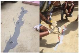
The system comes with a port, which is to be secured to the receiving substrate by means of KISEPO 10, and a spring-loaded injection device capable of up to 4-bar pressure.
